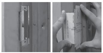
**2.** Peel adhesive backing and paste the folded template square to the frame.
