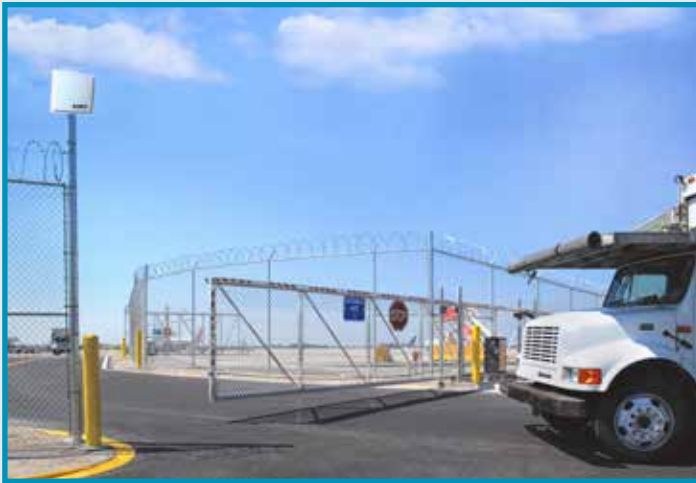
AVI (Automated Vehicle ID) Long Range Vehicle Tag System is adjustable from 8 to 25 feet.
