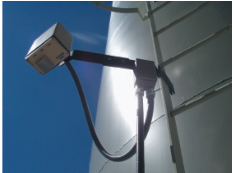
Front view of PH-6JB mounting bracket and junction box.
