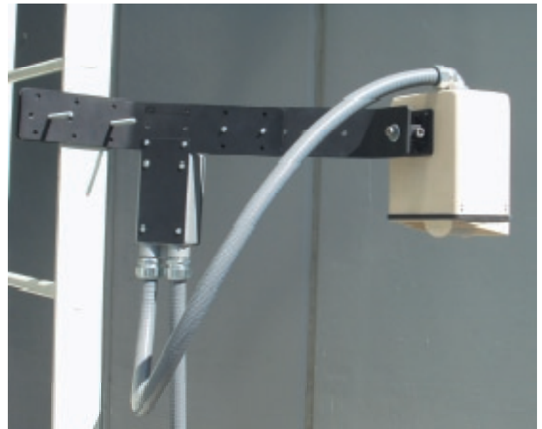
Rear view of PH-6JB mounting bracket and junction box.
