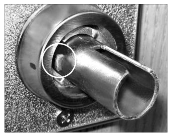
FIG. 6: PUSH IN LEVER CATCH (CIRCLED)
