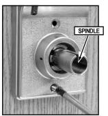
FIG. 15: TIGHTEN THRU-BOLTS
