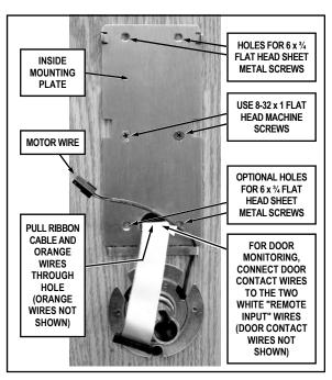
FIG. 13: INSIDE MOUNTING PLATE INSTALLATION
