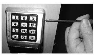
FIG. 17: SECURE THE TOP OF THE SECONDARY HOUSING
