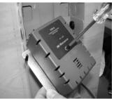
15. Insert and tighten the wires in the appropriate positions of the 4 position wiring connector (if provided) on the back of the new detector.
