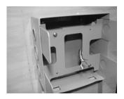
11. Push the adaptor all the way to the back of the box. The adaptor can be tapped with the butt of a hammer handle to be sure that it is seated all the way down into the box. Make sure that the wires are not pinched.
